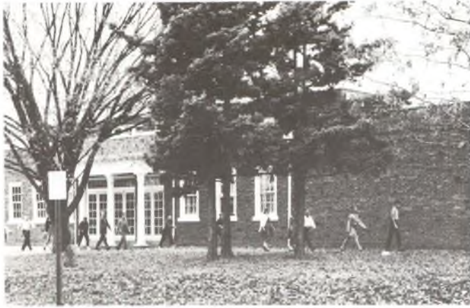
Glenmont Elementary School 1926
