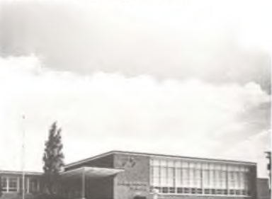
Cedar Grove Elementary School 1960
